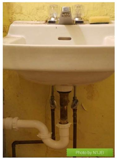
The second floor sink drain literally corroded away from the cast iron vent stack on the second floor of the club a month ago and began to leak thru the ceiling of the first floor.
