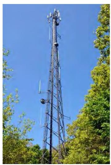
Our system utilizes two antennas. As pictured, ours are the thinner ones on the left of the tower. The bottom antenna, just below the left microwave dish is the transmitting antenna while the receiving antenna is near the top of the tower, positioned directly above the bottom antenna for the greatest signal attenuation.
