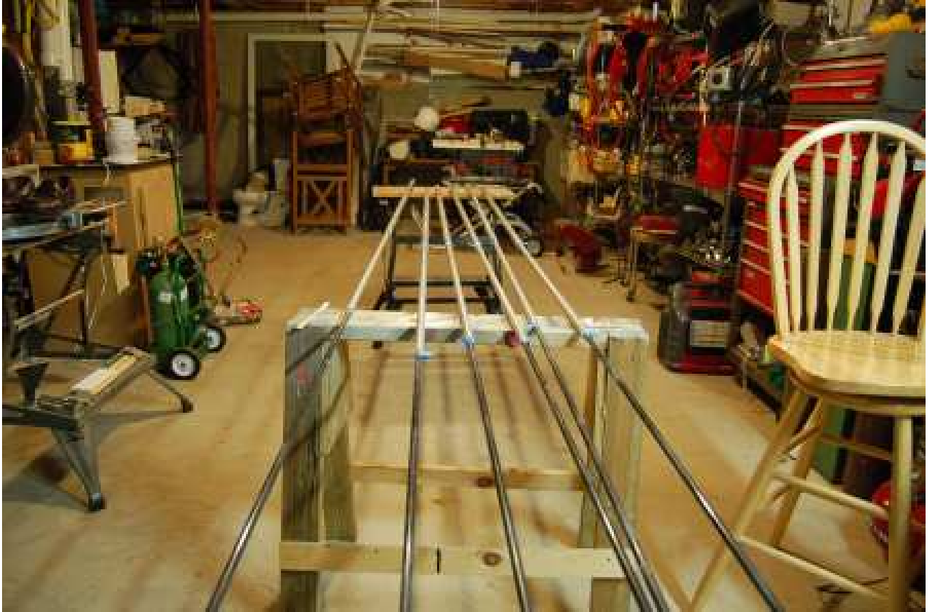
The fiberglass poles glued together before I primed and painted them. It is important to paint fiberglass as it will breakdown in sunlight in a short period of time. PVC is not a good alternative for the spreaders but many use Fishing Poles with good results.
