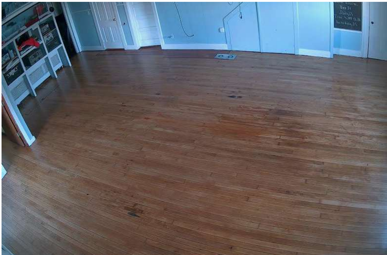
The finished job with 3 coats of polyurethane
