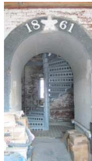
Inside the South Lighthouse
