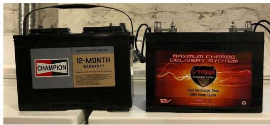
sizes. Don't forget to get a "DEEP CYCLE" type of battery as you will get a longer time of discharge thus a longer run time on your ham radios One last thing. Please use only a AGM type battery charger on AGM batteries since they need a higher voltage to recharge properly since they are built to recharge faster than the cheaper flooded batteries. I will show you next month a NOCO battery charger that I am using. That's it for now. See you next month!
